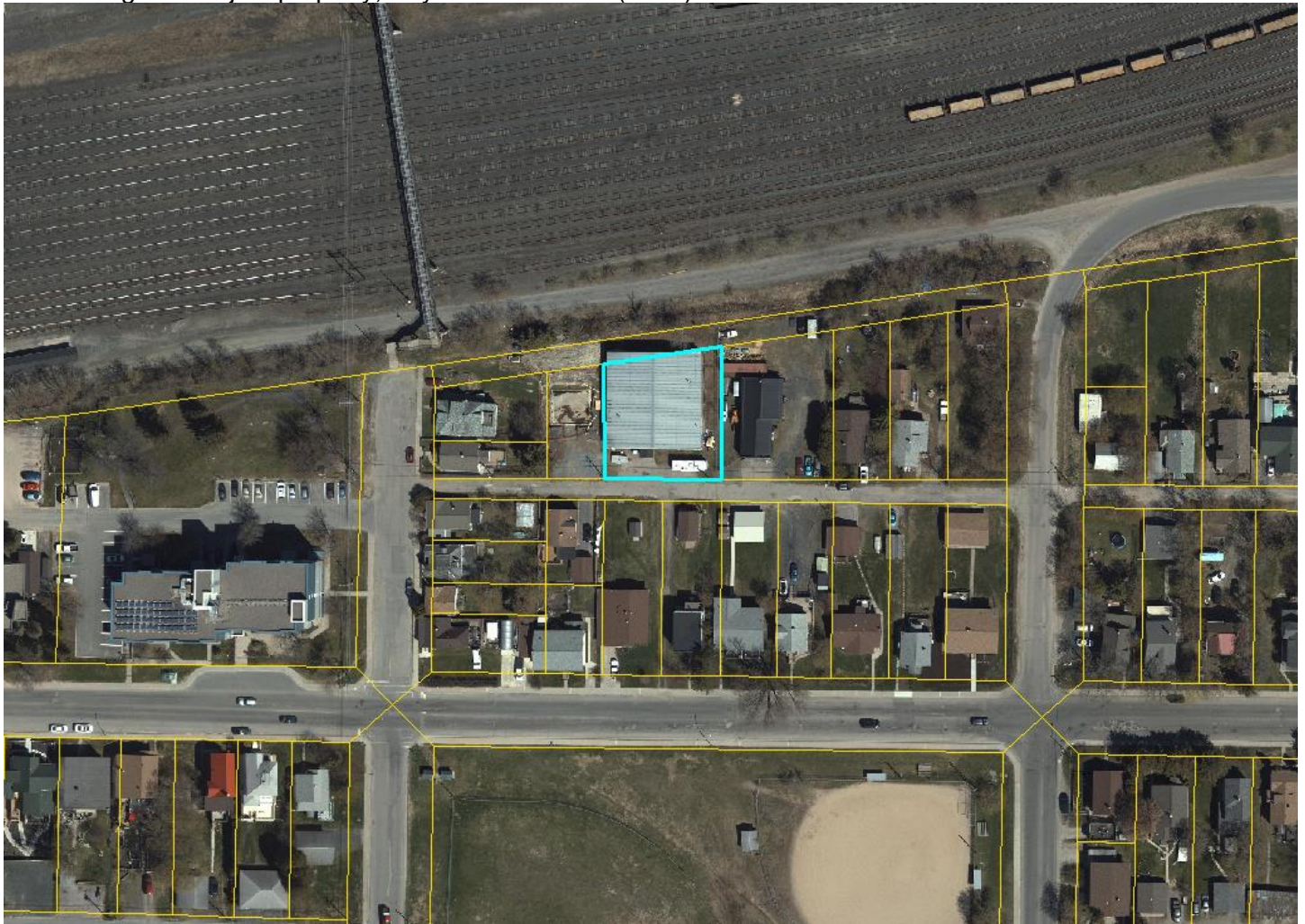
Aerial image of subject property, City of Kenora GIS (2019)
